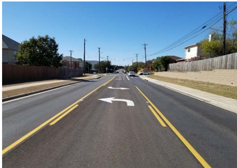
A completed street from the 2019 Street Improvement Program.
