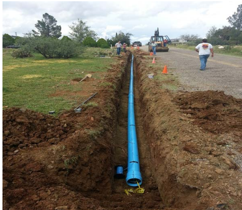
An example of a waterline installation.
