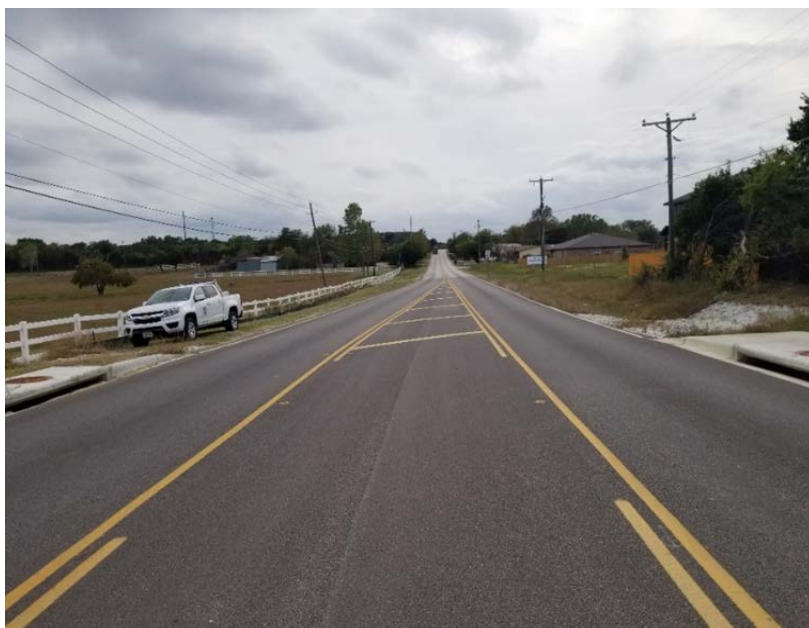
Completed portion of Warrior's Path Phase 1. Phase 2 will go from Pontotoc Trace to FM 2410/Knight's Ridge.
