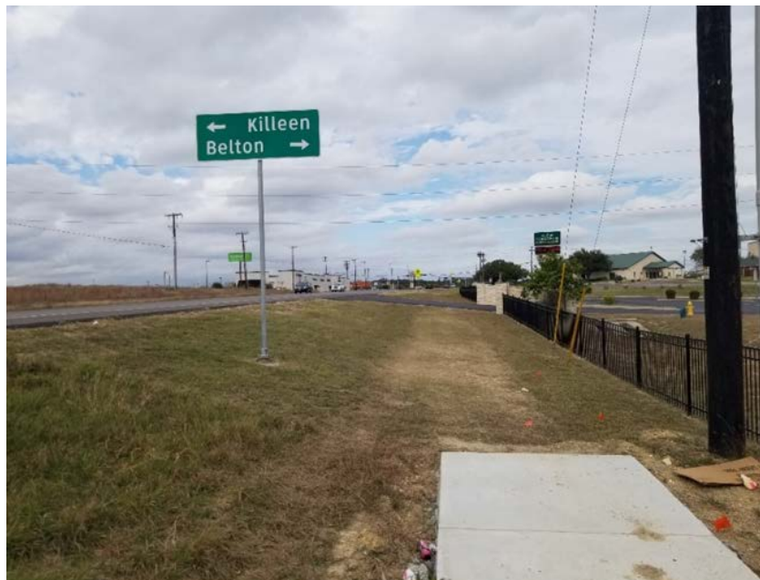
Construction area for the FM 3481 Sidewalk - Phase 1.
