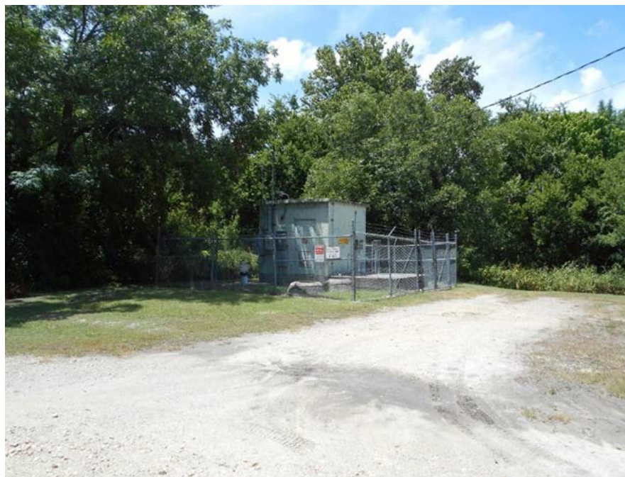
VFW Lift Station Wetwell
