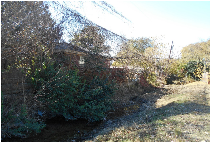
Picture of where the concrete retaining wall will be placed.
