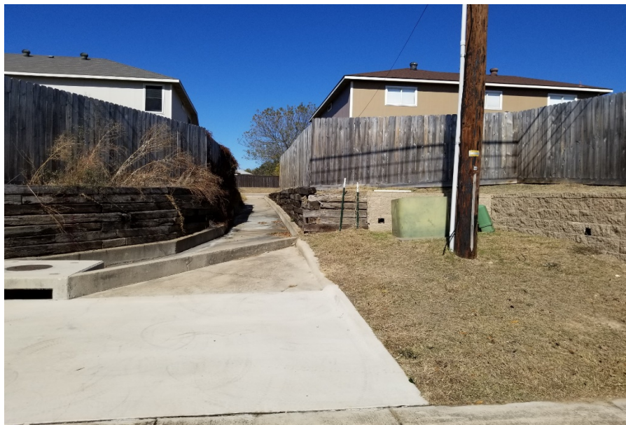
Site of the Drainage Flume Reconstruction Project.
