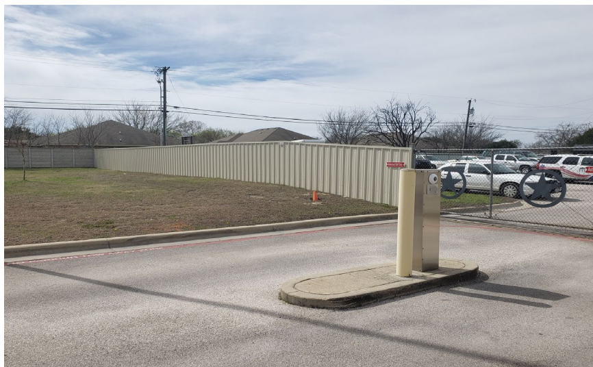
The new metal fencing installed at the Police Station
