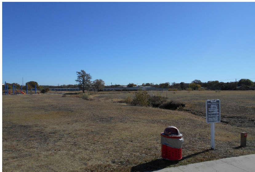
A look at the current Goode-Connell Park water detention facility.
