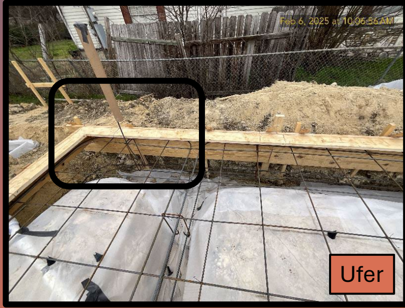
Sleeve through foundation wall
